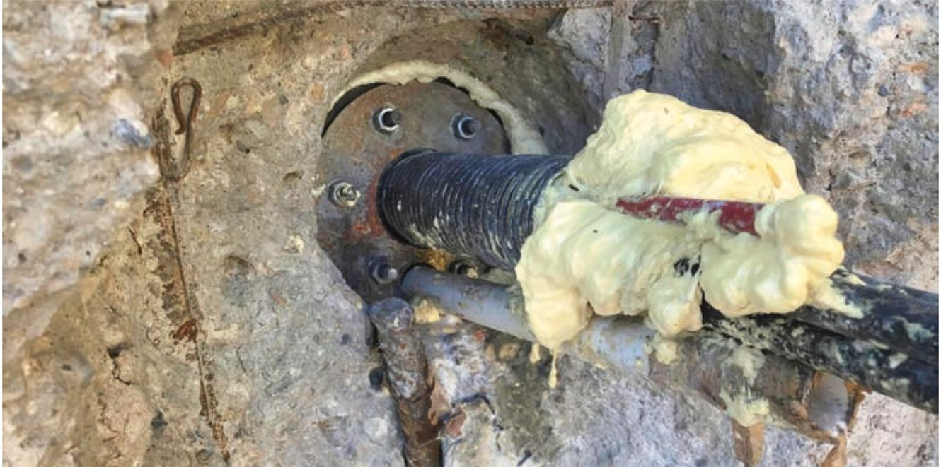
Injection for sealing on an anchor head
