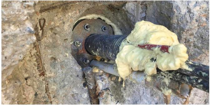
Injection for sealing on an anchor head
