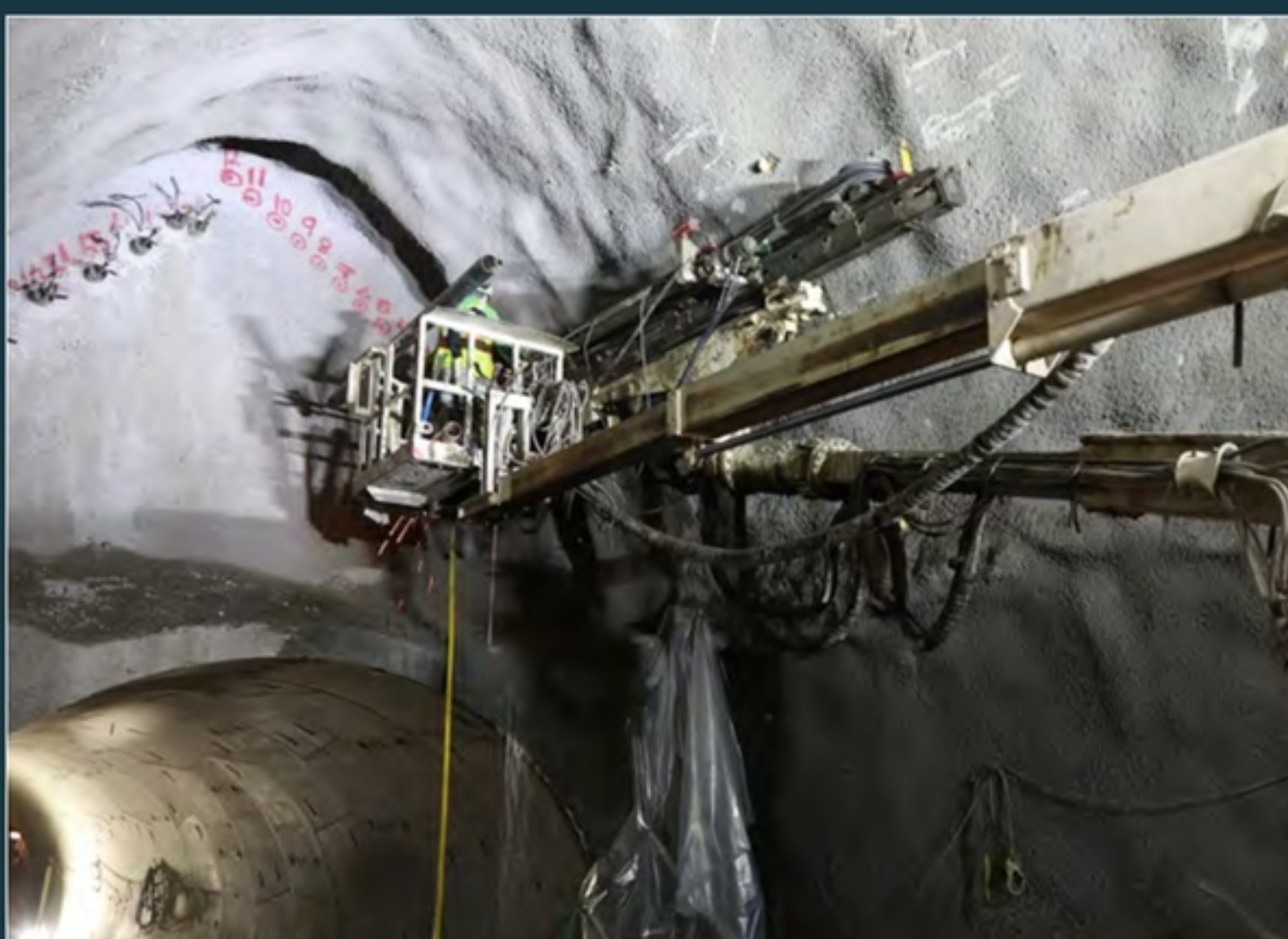
The Austrian invention has spread to North America. Here is Eglinton Line Toronto, which used DSI's AT Pipe Umbrella System 2019.
