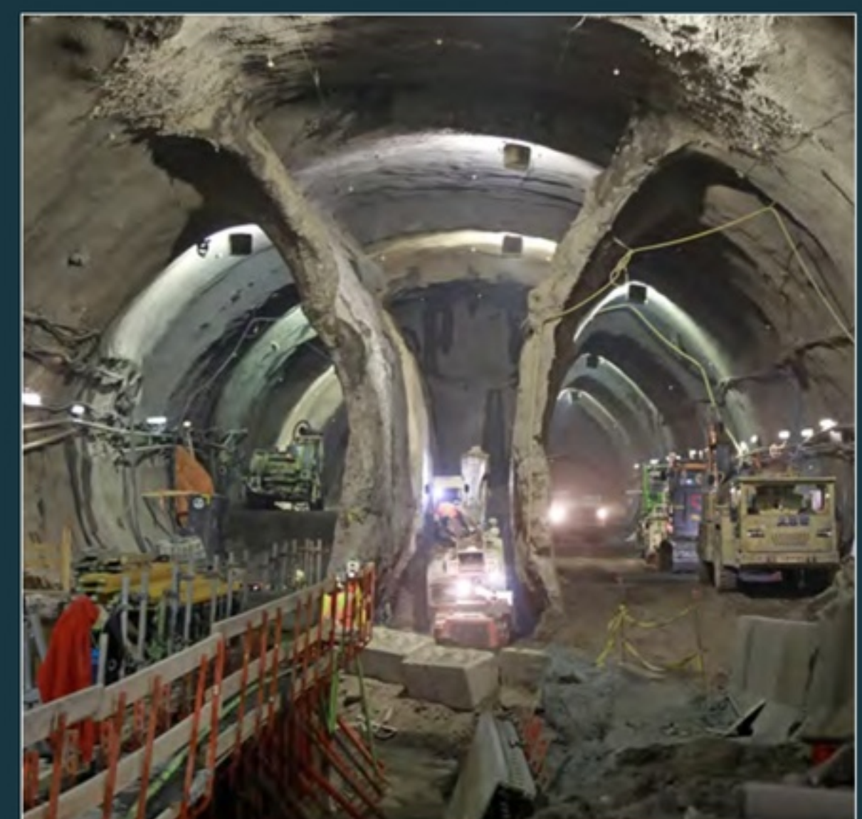
The Austrian invention has spread to North America. Here is Eglinton Line Toronto, which used DSI's AT Pipe Umbrella System 2019.
