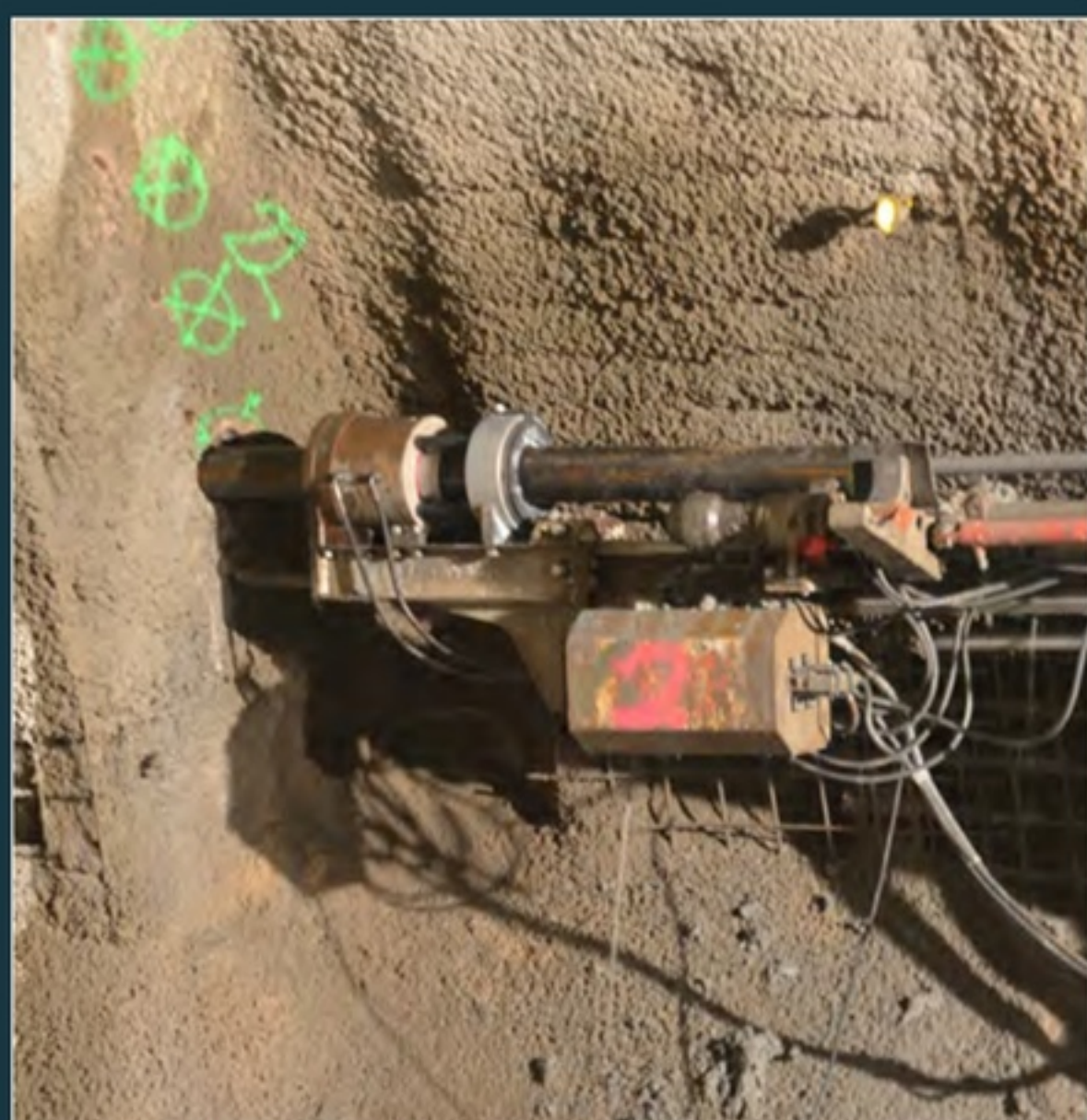
Germany's Hirschhagen Tunnel was the first to use squeezing joints in 2015.
