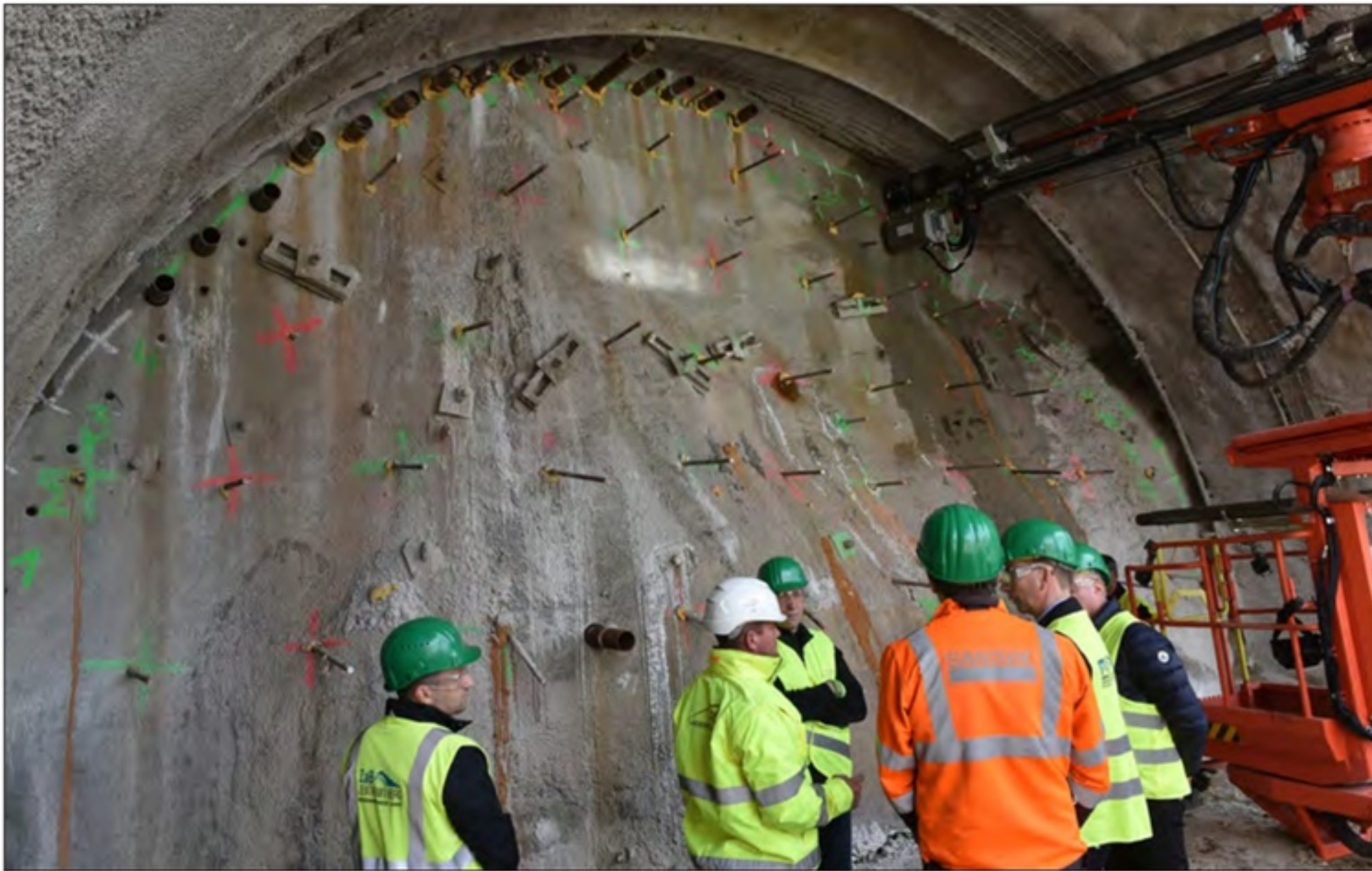
Full-scale demonstration at Montan University Leoben's Zentrum am Berg.
